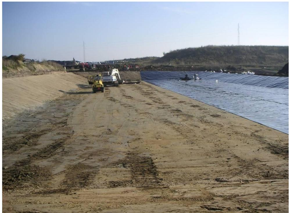
Figure 28 Construction of clay liner and installation of HDPE-liner
