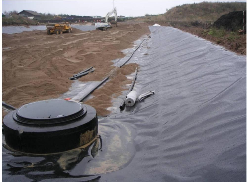
*Figure 29 Installation of drainage layer on top of the HDPE-liner*
