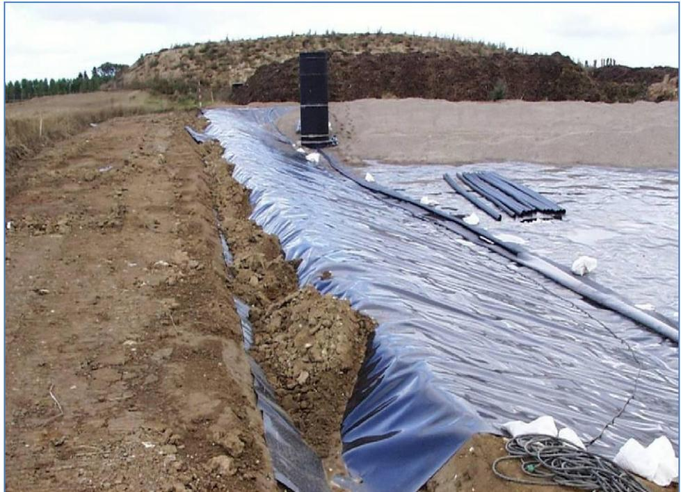
*Figure 30 Construction of waste disposal cell, with bottom clay layer, HDPE liner on bottom and slopes, and a leachate collection well at the lowest point of a landfill cell*
