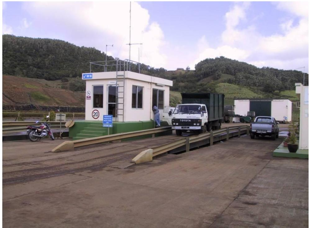
Figure 31 *Electronic weighbridge for trucks delivering waste to the landfill*
