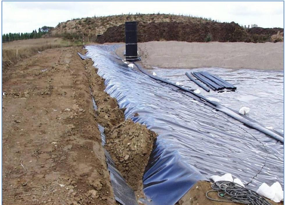
*Figure 30 Construction of waste disposal cell, with bottom clay layer, HDPE liner on bottom and slopes, and a leachate collection well at the lowest point of a landfill cell*
